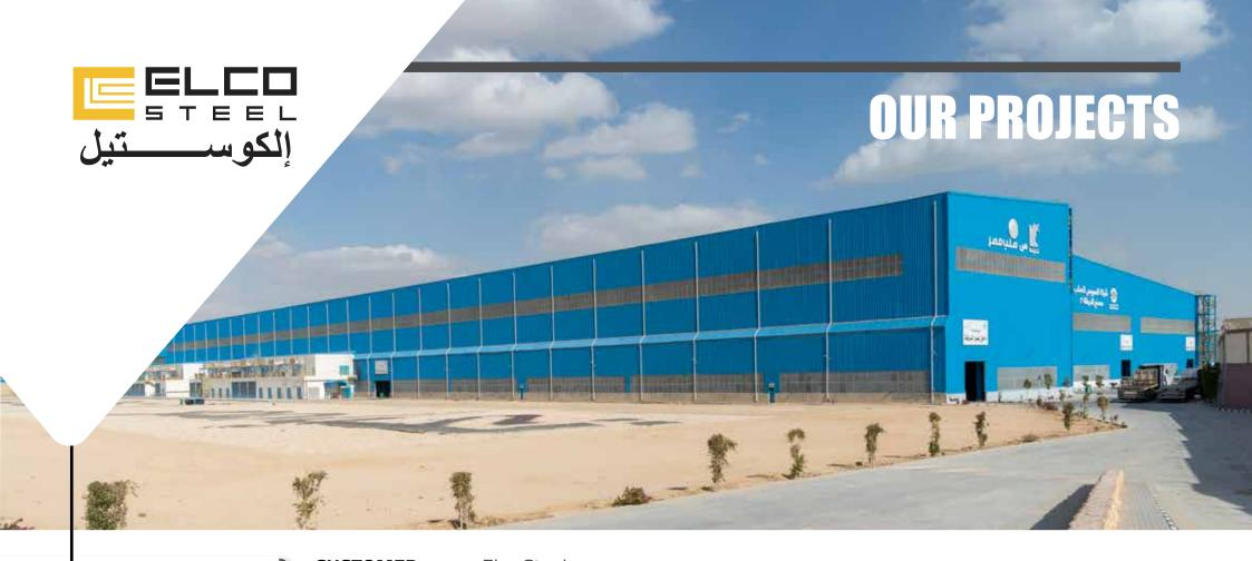
CUSTOMER: Elco Steel.DESTINATION: Suez City - Attaka.SCOPE: Supply, Fabrication and Erection of Rolling Mill Plant.DESCRIPTION: 8000 Ton of Steel Structure & Cladding Works.CONTRACT YEAR: 2017-2018
